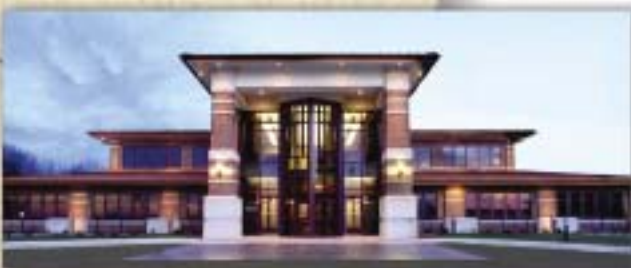
IMEA's current headquarters building, opened in 2007, reflects the style of the Prairie School of architecture championed by Frank Lloyd Wright. It encloses 33,000 square feet on three levels and was designed to meet the Agency's needs for 50 years.
