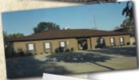
The IMEA headquarters on Conifer Drive was constructed in 2007. The building earned a U.S. Green Building Council Leadership in Energy & Environmental Design Silver Certificate, the first structure in Springfield to do so. The building was designed to use 40% less energy than would a conventional building of its size. It features geothermal heating and cooling, Solatube sky lighting and a tight building envelope that exceeded the then-existing building code requirements by 16%.
